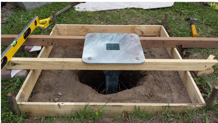
Appropriate hole with formwork and base elevated approx 240mm above ground.
