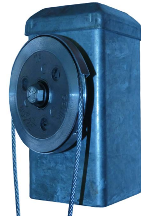
6. Pulley wheel retaining bolt tightened to retain winch cable
